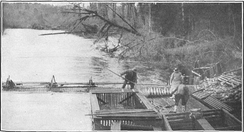
FIG. 41.—CHEHALIS HATCHERY, WASHINGTON FISH AND GAME COMMISSION, SHOWING RACKS TO PREVENT SALMON FROM GOING UPSTREAM, AND PEN FOR HOLDING SPAWNING FISH.
