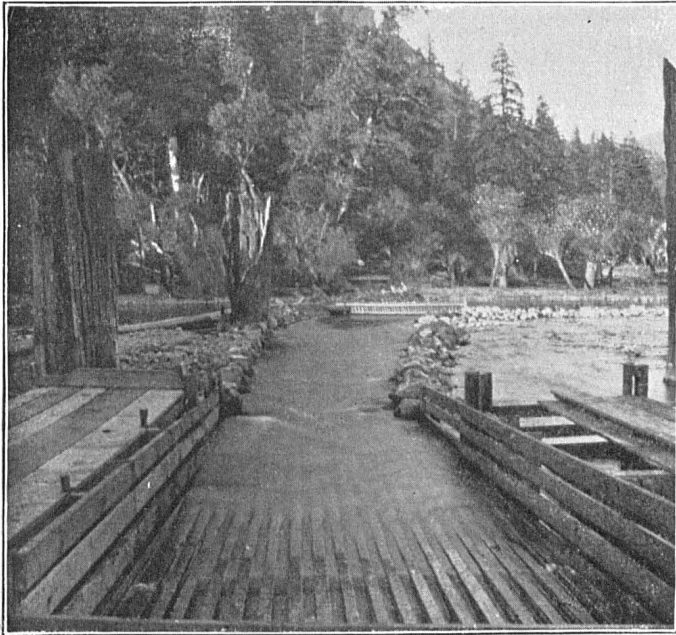
SALMON-PENS AND RETAINING-RACKS AT LITTLE WHITE SALMON STATION.
