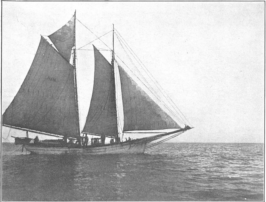
A DREDGING VESSEL AT WORK, PAMLICO SOUND.
