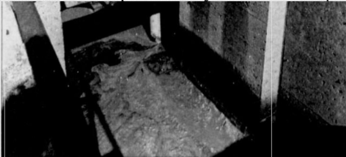
Workers from Clean Harbors Environmental Services Inc. use machinery to suck up fuel-laden muck from a weir at General Alum and Chemical Corp. in Searsport, which owns the concrete catch basin containing the gunk. The operation was overseen by the U.S. Coast Guard, which required the cleanup. (NEWS Photos by Bob DeLong)
