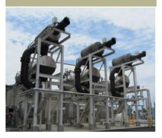
to integrate with the CHP system. Woodard & Curran and the client chose a steam turbine chiller with existing HVAC controls to meet the goals of the facility. The chiller also utilizes the environmentally conscious R-134a refrigerant to ensure the chilling process is as efficient as possible.
