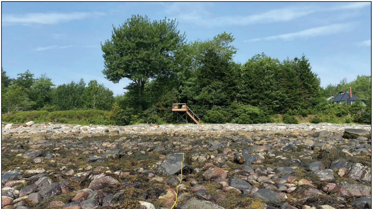
Photograph Two. Facing westerly – view of existing structure that provides access to intertidal area. Photographer: Tim Forrester, Atlantic Environmental, LLC Date: July 16, 2021.
