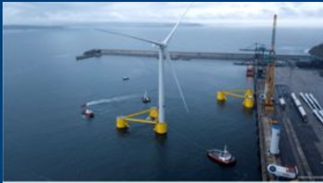
WTG Installation at Berth
