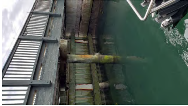
Photo 11: End of Jetty
