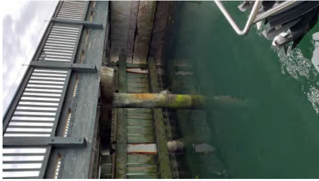
Photo 11: End of Jetty
