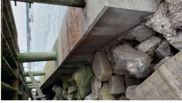
Photo 13: Beginning of Pier
