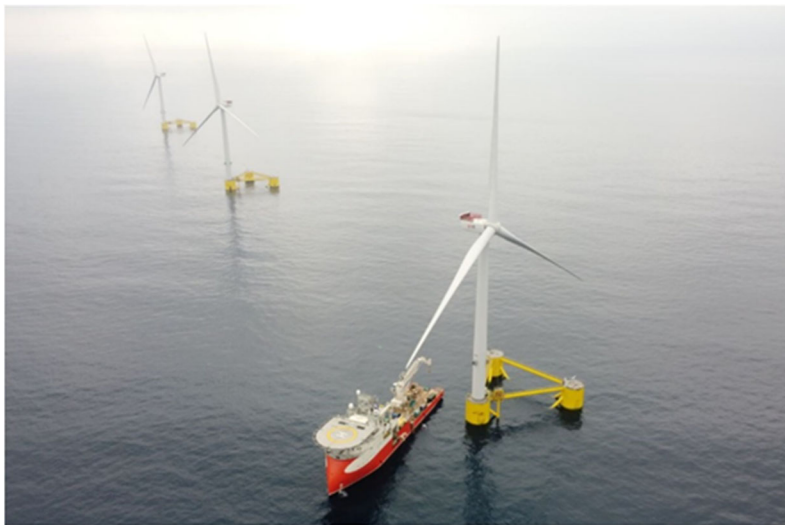
Figure 3-1: WindFloat Atlantic Installation (Source: EDP Renewables)
