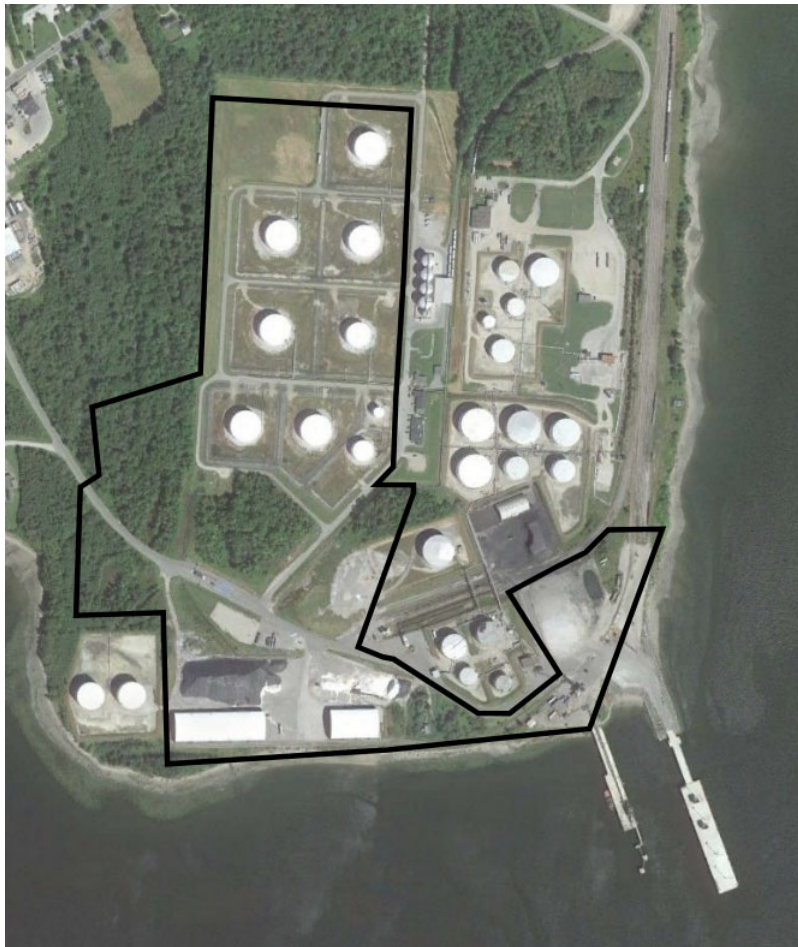
Figure 5-1: Available Area at Mack Point Terminal
