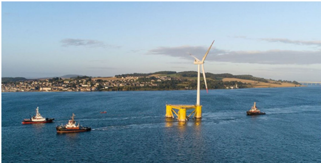
Figure 3-2: Completed Kincardine Floating Turbine Being Towed to Installation Site (Source: Cobra Group)
